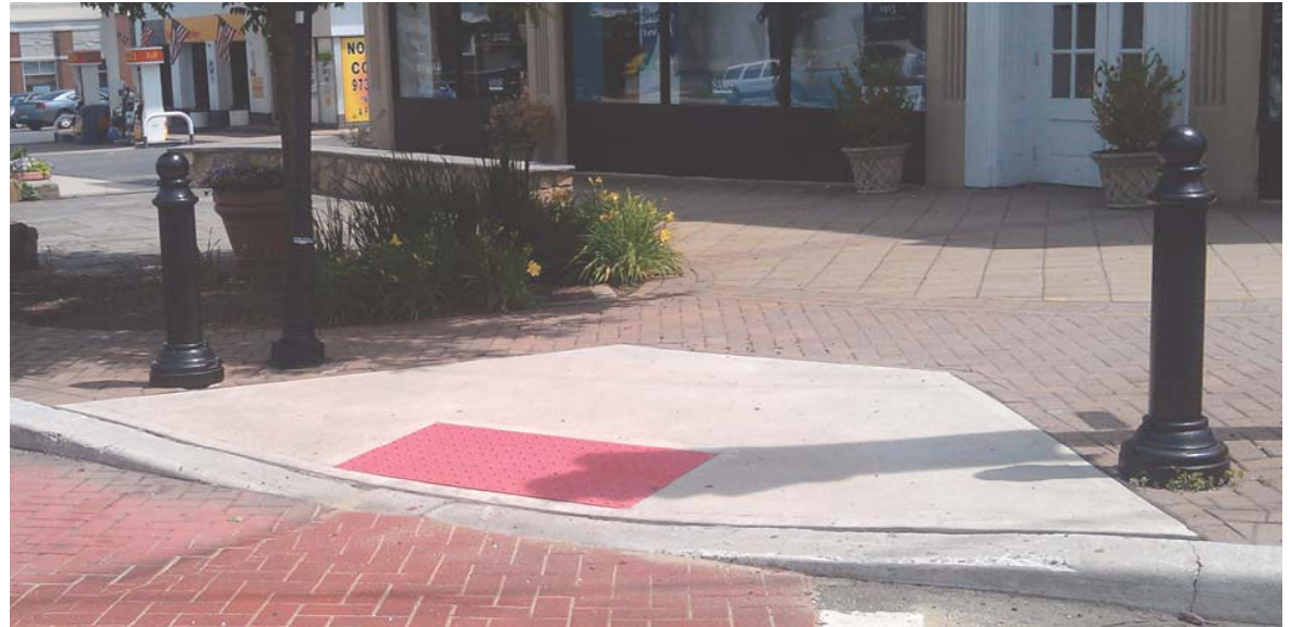
Protective bollards at the corner
