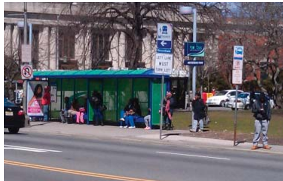
Covered NJ Transit GO Bus Stop near the Post Office in Bloomfield
