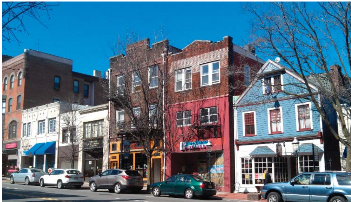
Existing downtown storefronts along Bloomfield Avenue in Montclair Township
