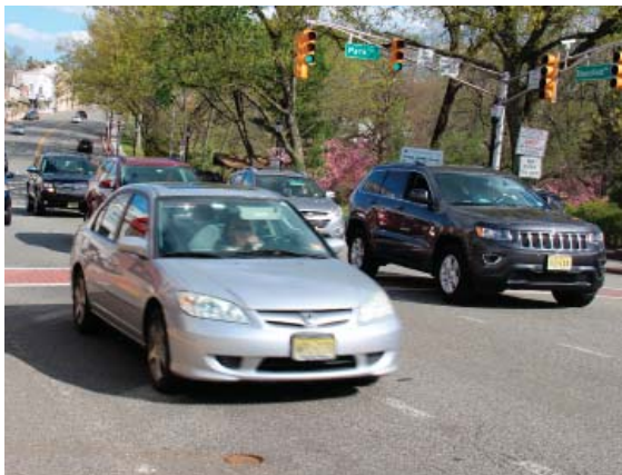
Faded lane guidelines cause vehicles to drift into adjacent lanes
