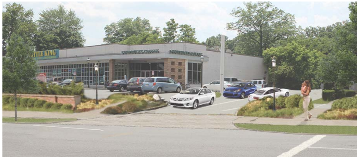
Photo montage of consolidated curbcuts
