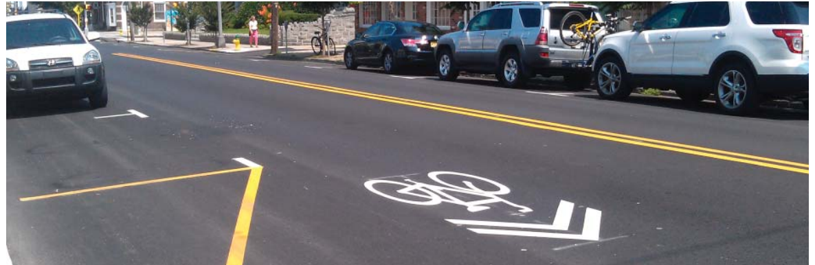
The bike network should be coordinated amongst the towns and the County and include a combination of dedicated bike lanes, sharrows (share the road markings), and off-street trails.
