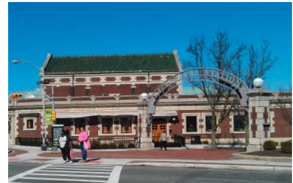
Pedestrian plaza and curb extensions at Lackawanna Station in Montclair
