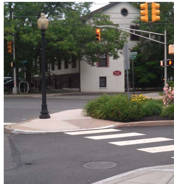
The existing painted pedestrian shelter island can be with raised curbing and plantings
