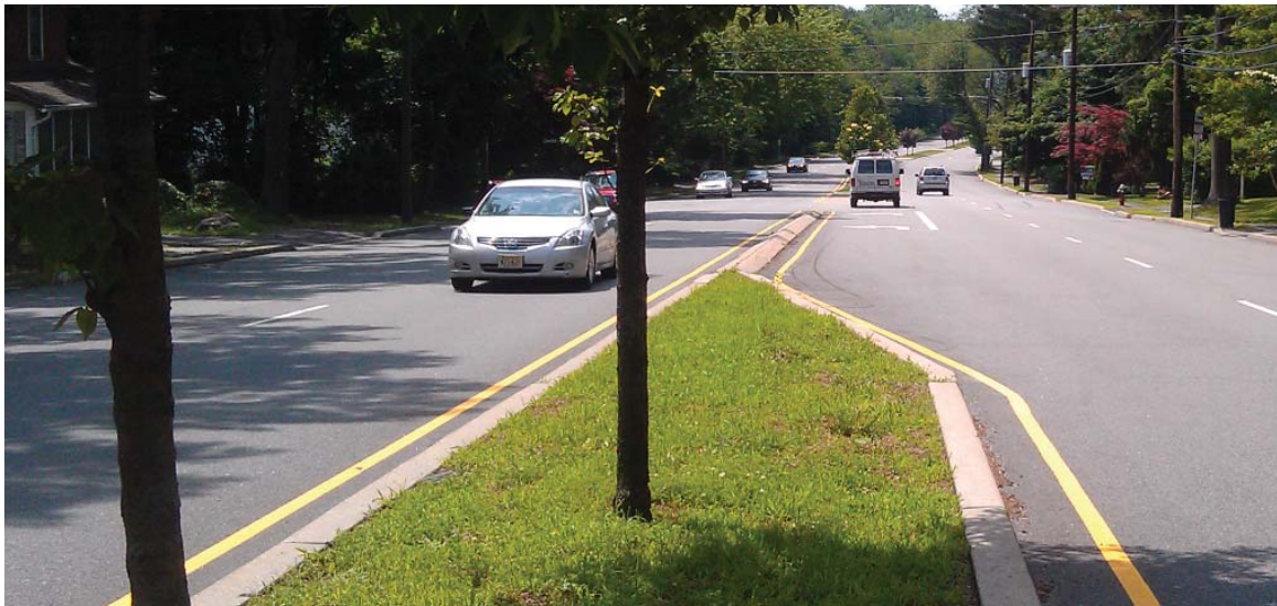
Planted median along Northfield Road (Essex County Rt. 508) in Livingston, NJ
