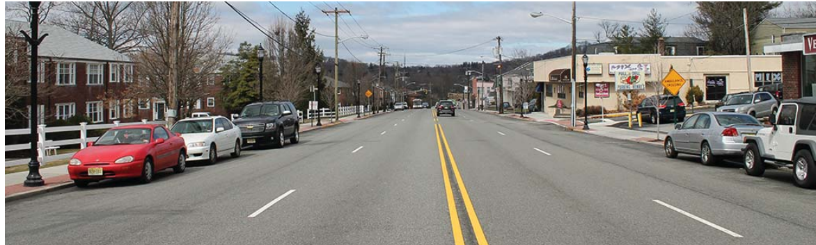
Unmarked parallel parking and four travel lanes on Bloomfield Ave near Church Street in Verona. The perceived road width can encourage higher speeds in some areas in the corridor.
